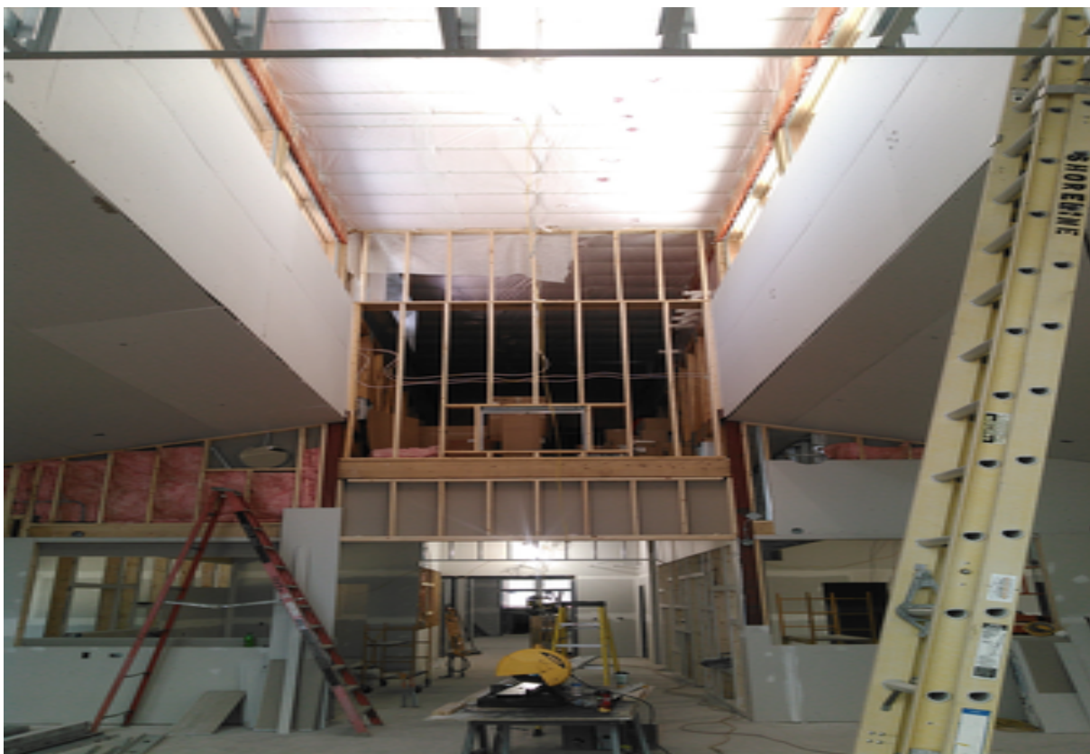
Finishing drywall in Clerestory
