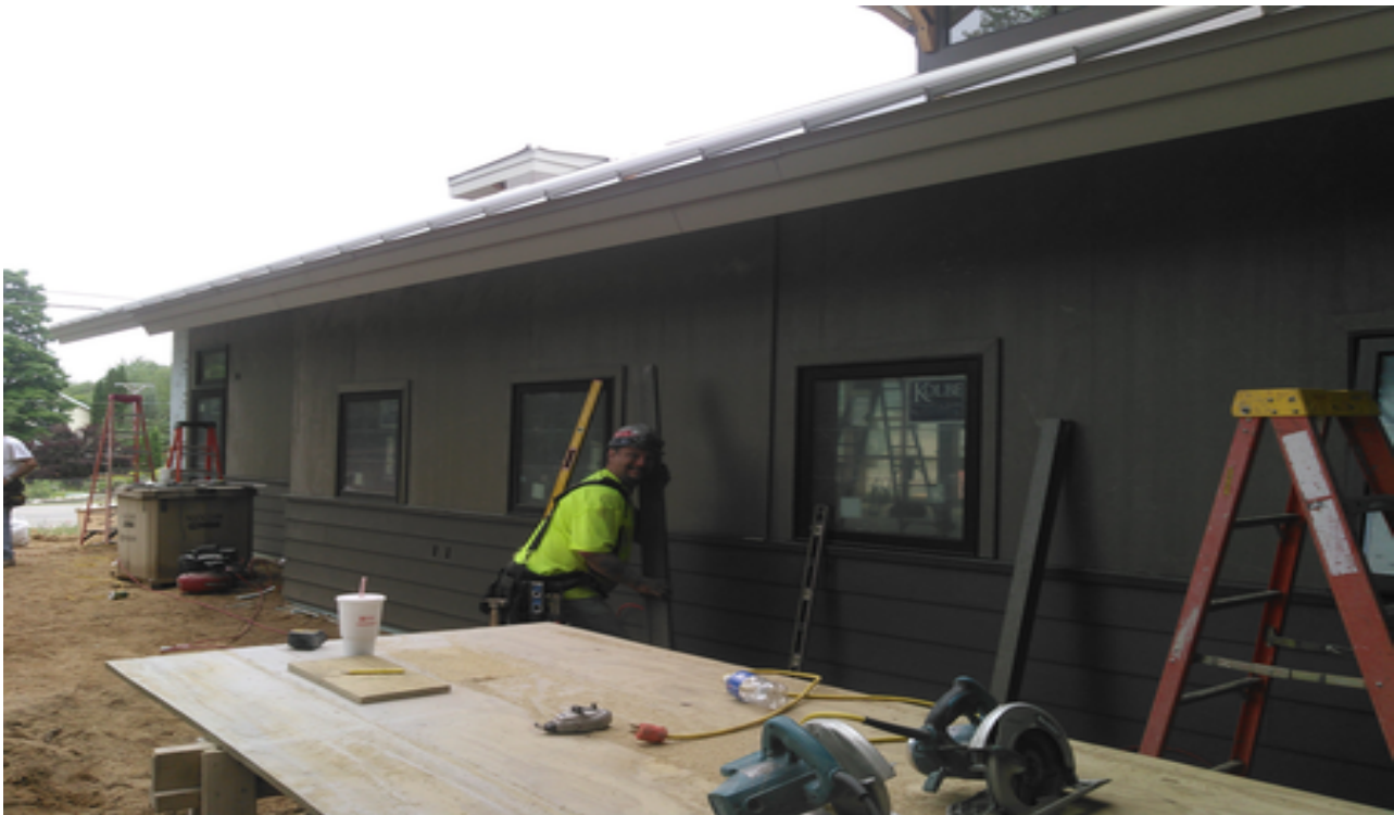
Installation of siding on Study Room Walls
