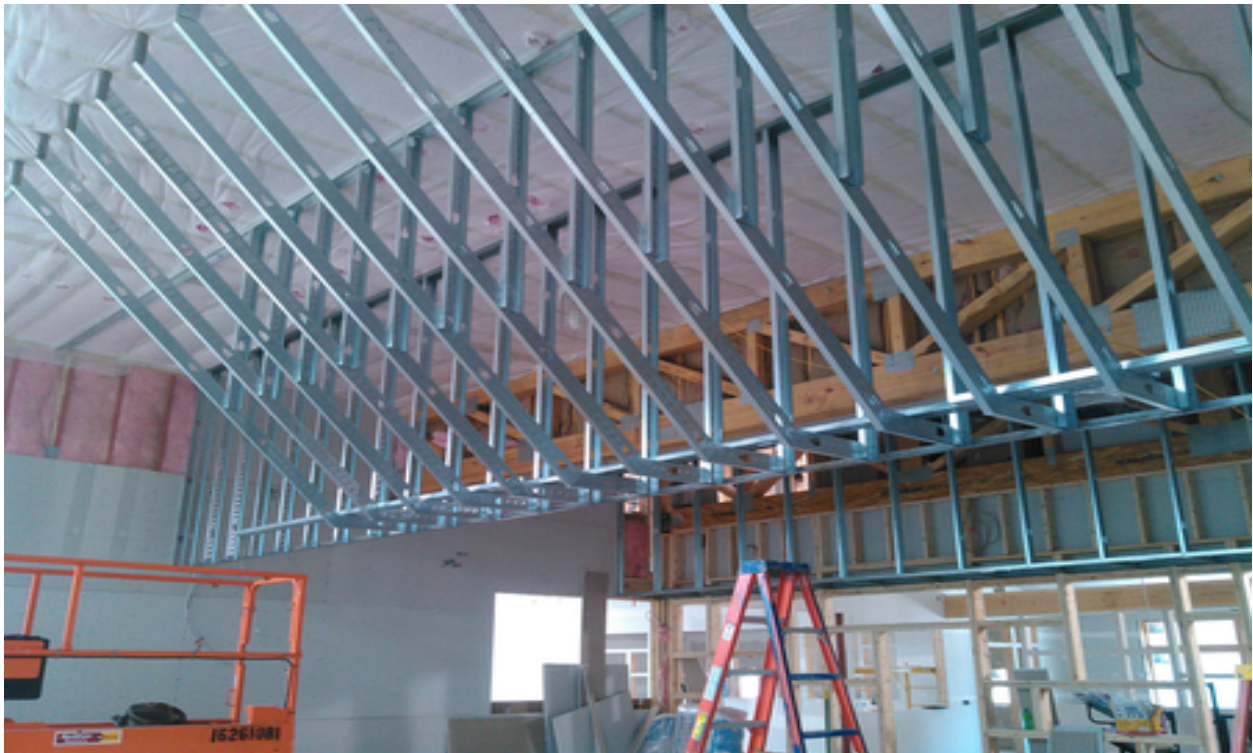
Framing up bulkheads
