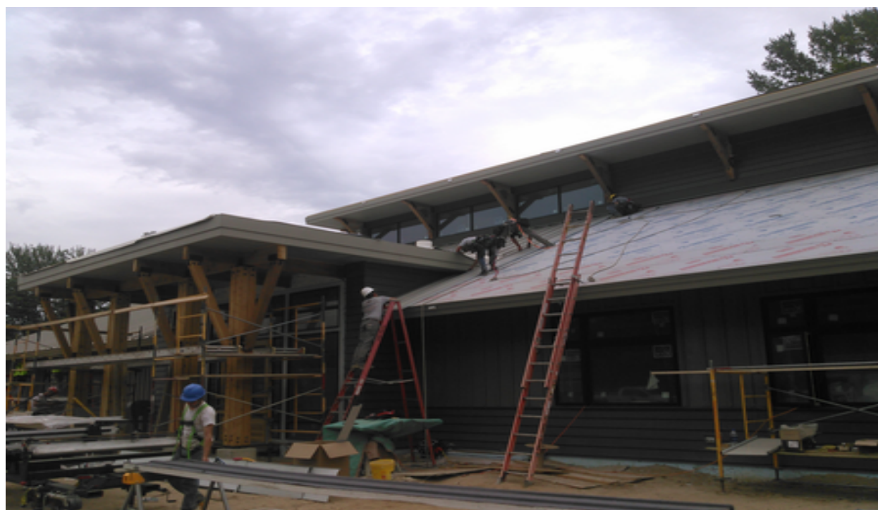
Metal roof installation on north side of building
