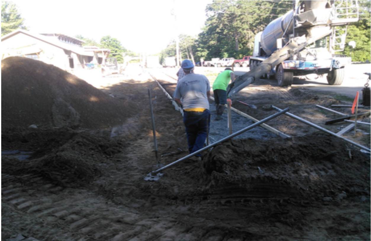
Framing up bulkheads
