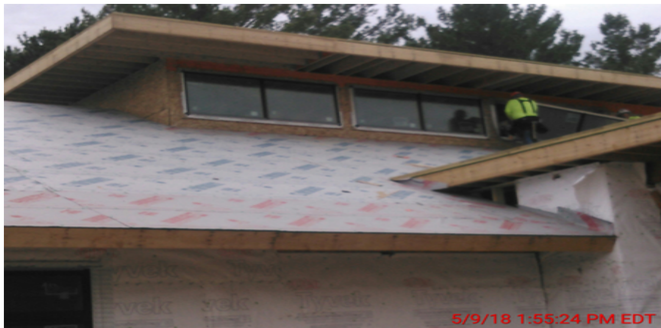
Installation of Clerestory windows
